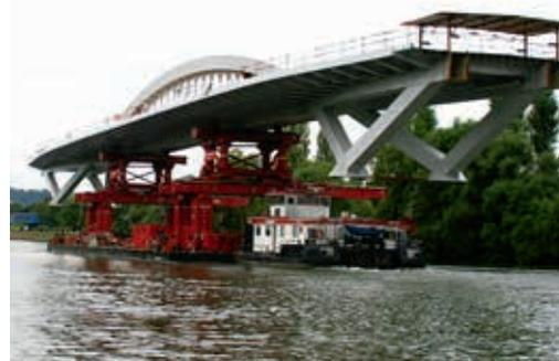
Transport of the bridge's central span by lighter along the Moselle.
